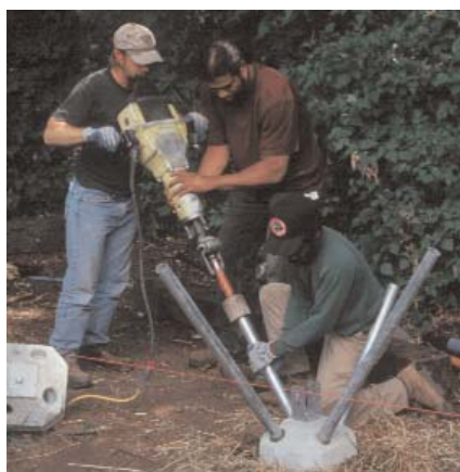
DP-100, Diamond Pier w/ 6x6 Post Attachment
